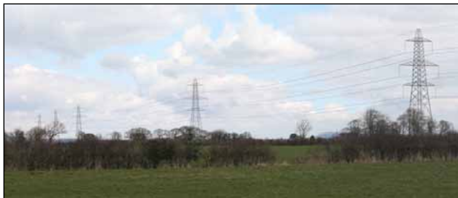
Existing L6 Tower
