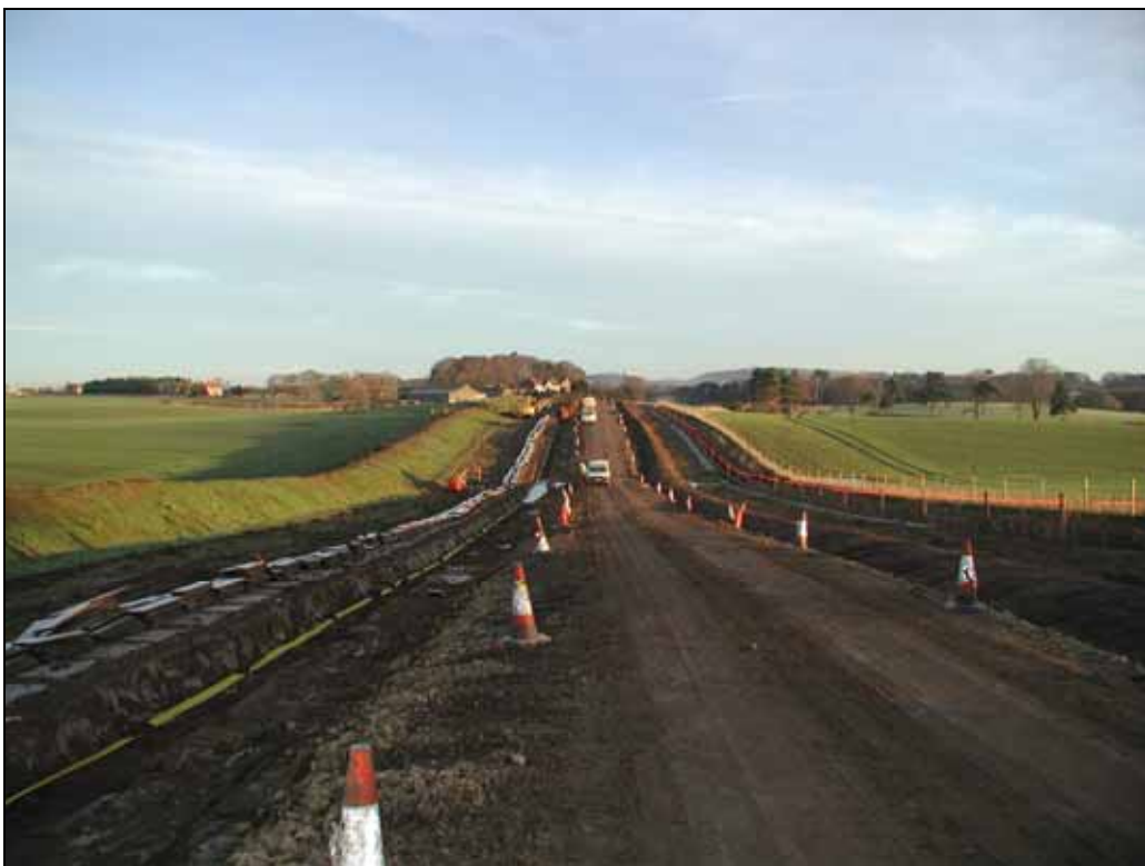
Figure 5.9 Construction Working Area during Underground Cable Laying
