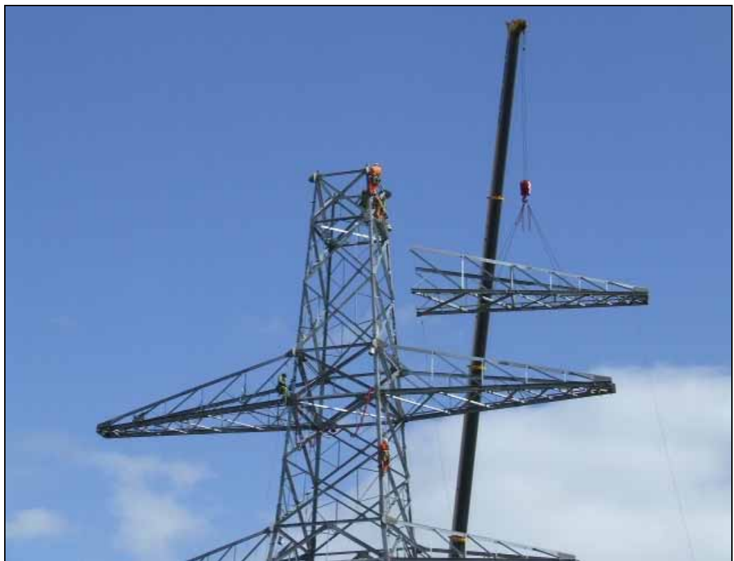
Figure 5.6 Crane Assembling a Tower
